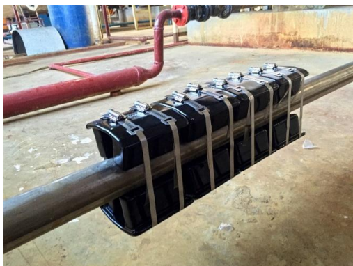
Figure 3: GMX8000 installed on a boiler gas line (side view)
