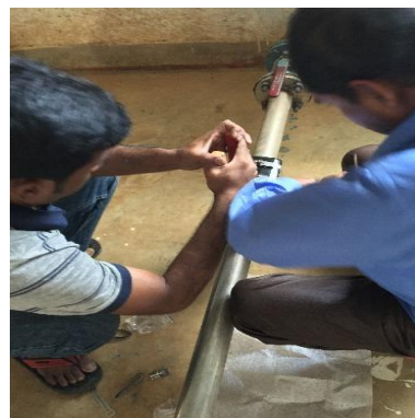
Figure 4: MS pipe replacement with SS pipe
